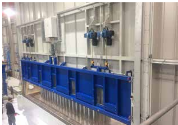
TOP: GALVANISING PLANT LIMBACH BOTTOM: GALVANISING PLANT OELSnitz
